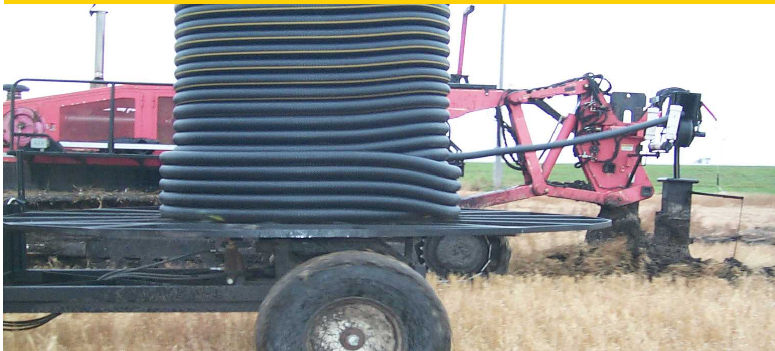
Figure 8. Installation of tile drainage in progress in Ramsey County along state Highway 17 near Edmore, N.D. (Photo courtesy of Ronald Beneda, NDSU Cavalier County Extension agent).
