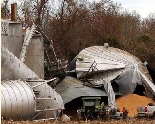
Bridging transfers load to the bin wall
