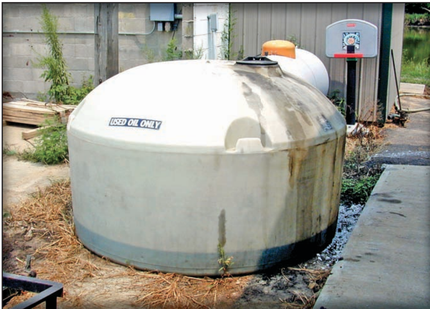
This tank would not pass a regulatory inspection.
