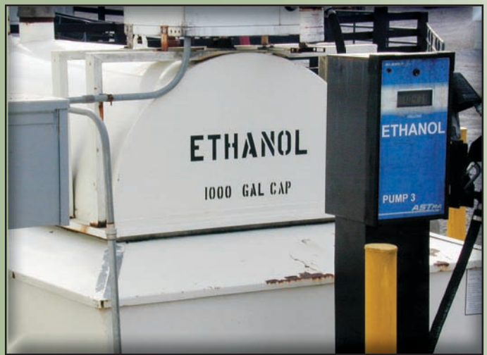
The tank capacity is stenciled on the exterior to help ensure against mistakes while loading fuel from the fuel truck.
