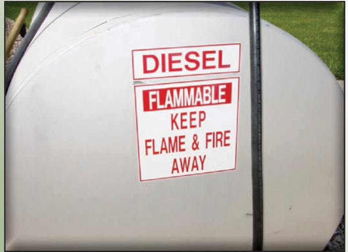
This tank is marked with large lettering indicating the product type and warning the user about hazards associated with the product.
