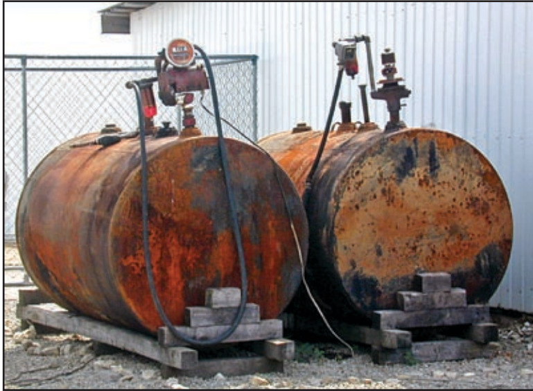
Above and right: These underground fuel tanks are being reused for aboveground storage. Notice the extreme corrosion in the right-hand photo. Tanks previously used underground should never be reused for aboveground fuel storage.
