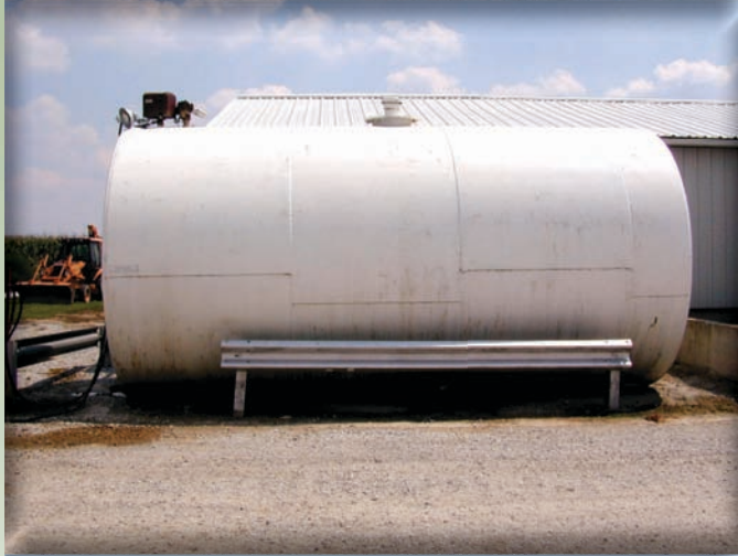
These are examples of barriers that protect fuel tanks from vehicles.
