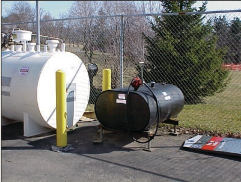
Above: The black indoor tank is being used outdoors.
