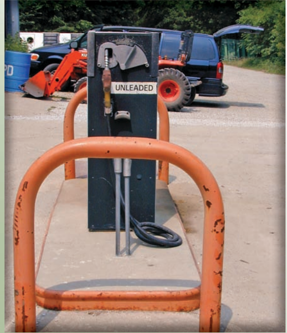
These are examples of barriers that protect fuel tanks from vehicles.
