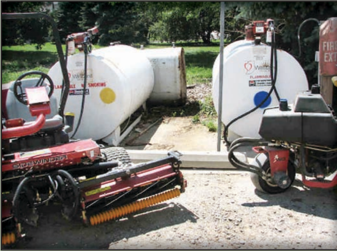
Fuel tank caps can be color-coded to match the tanks.
