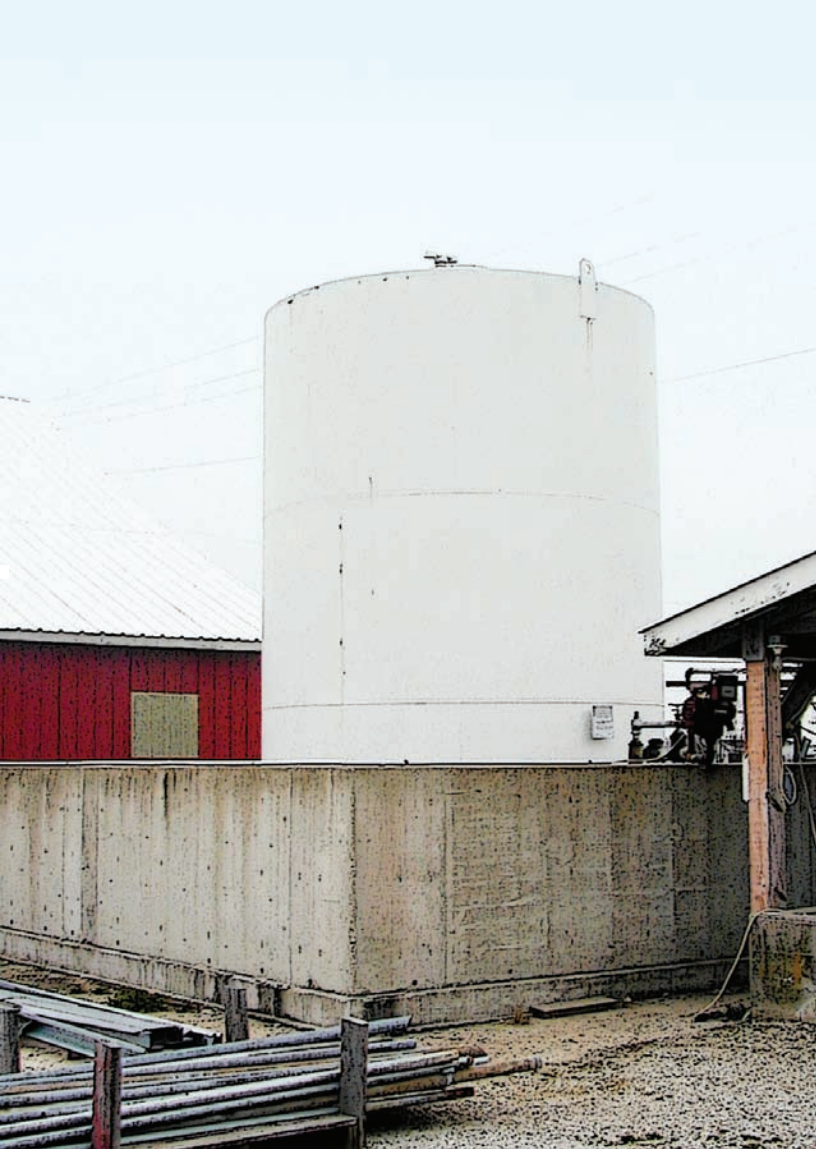
Above: Large diesel tank in containment.
