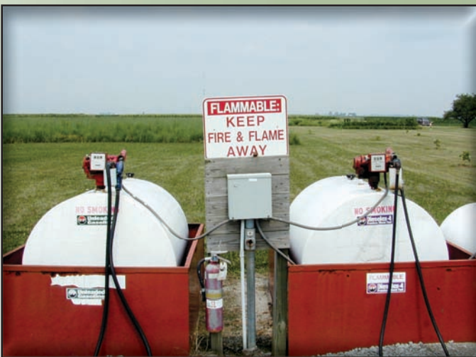
These tanks rest in rectangular metal dikes to contain spills. Hose nozzles are placed in rain bonnets. A fire extinguisher hangs nearby for handling accidental fires.
