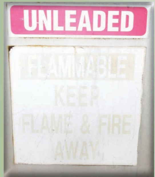
The labels on these tanks are faded and worn—some even partially torn off—making content identification difficult.
