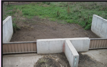
This properly functioning solid separator has been scraped of its solids.
