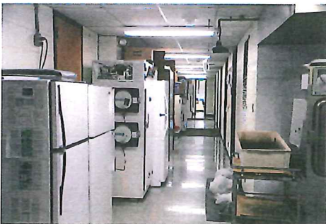
This third floor Walster Hall was designated a "room" so fire codes are not violated by equipment in the hallway. Equipment housed here is used daily.
