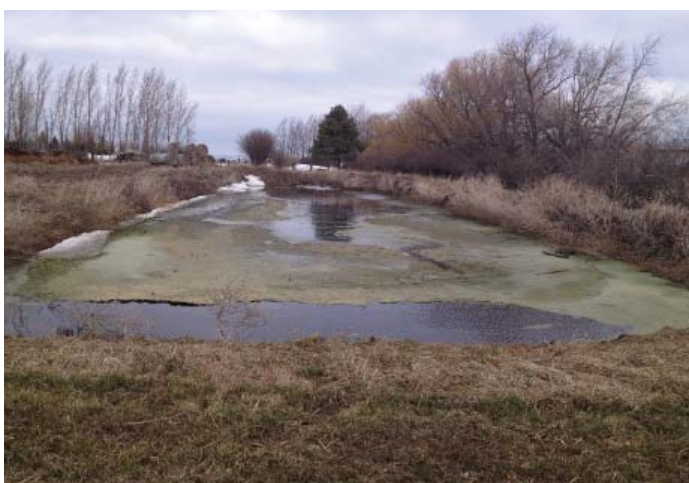
Figure 2. An effluent containment pond. Ponds are designed to hold water for a period of 270 days plus a 24-hour, 25-year rain event, while allowing at least an additional foot of freeboard.
