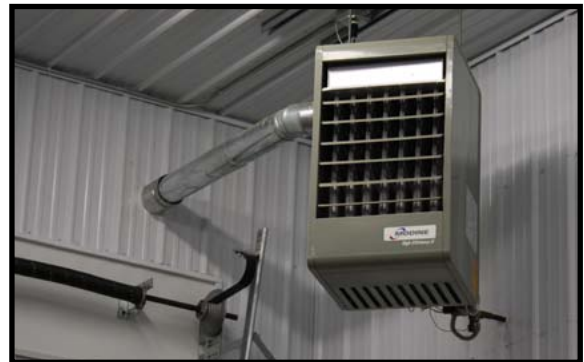
Figure 1. Forced-air propane furnace. (Carl Pedersen, NDSU)
