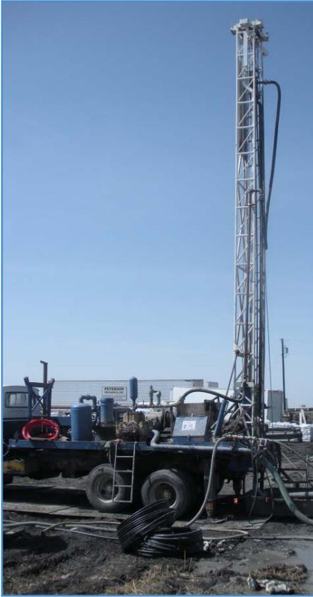
Figure 6. Drill rig installing vertical ground loop
