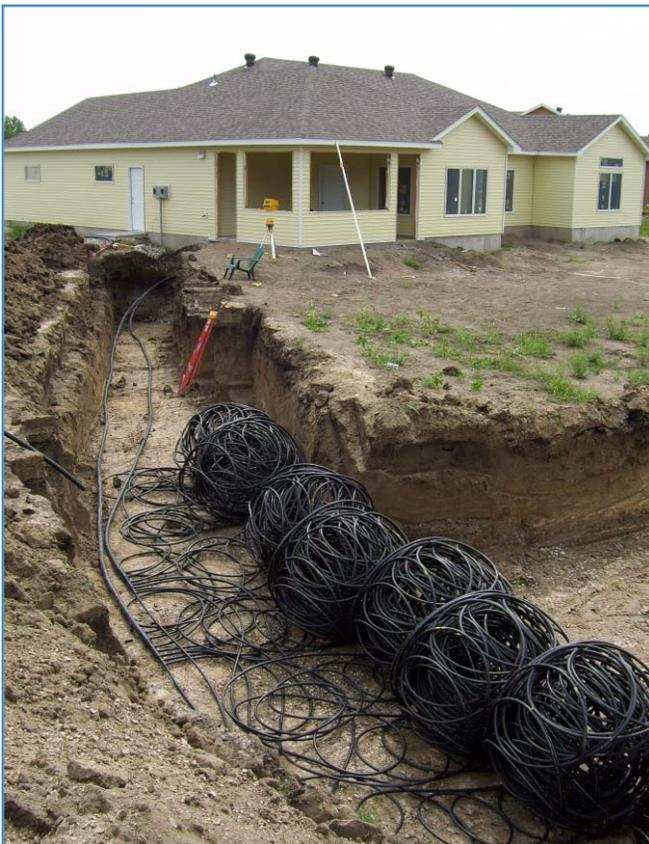
Figure 4. Horizontal “slinky” system installation (before)
