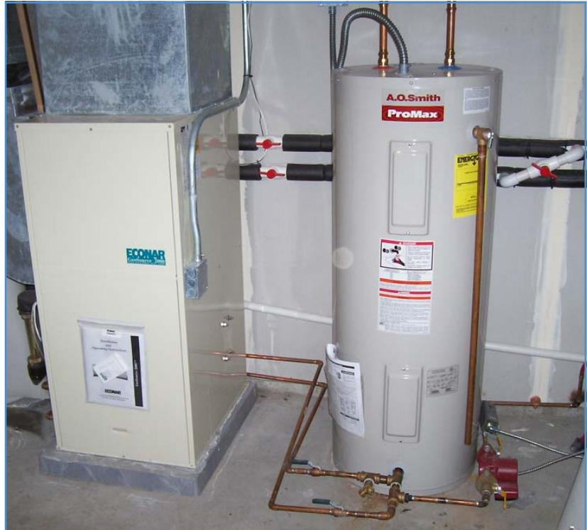
Figure 1. Forced-air heat pump with desuperheater.
