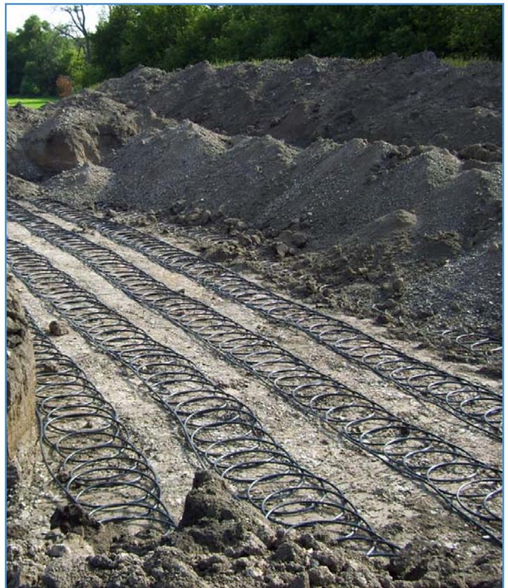
Figure 5. Horizontal ground loop (after)
