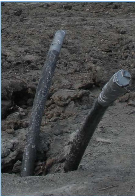
Figure 7. Installed vertical ground loop
