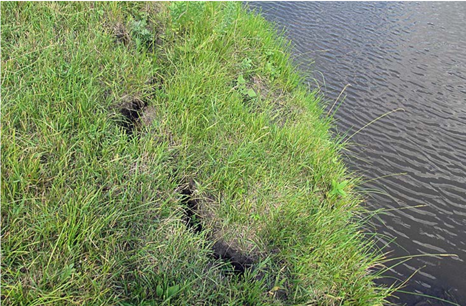
Tensile cracks on streambank where riparian species have been replaced by Kentucky bluegrass. (Miranda Meehan, NDSU)
