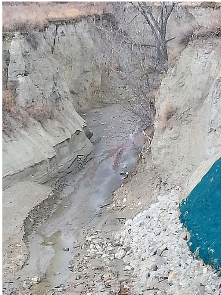
G streams are gully- or trench-shaped, being narrow and deep with no floodplain. (Miranda Meehan, NDSU)
