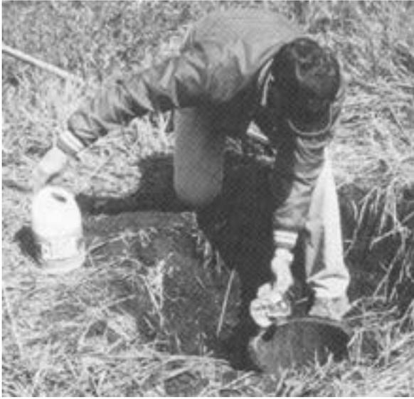
**The chlorination procedure disinfects the well so that disease-causing microorganisms are not sealed in the aquifer after the well is plugged.**
