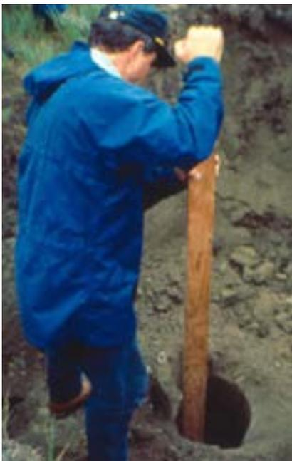
Tamping native clay as it is shoveled into the well is an important step to insure that all voids are filled and minimal settling will occur.
