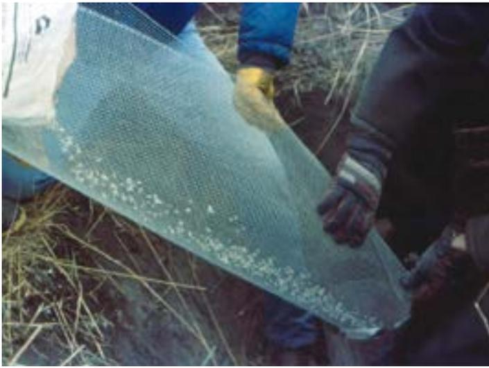
Because of the ease of application, chipped bentonite is the recommended material for plugging abandoned wells less than 10 inches in diameter. The bentonite chips should be poured slowly over a screen prior to entering the well.
