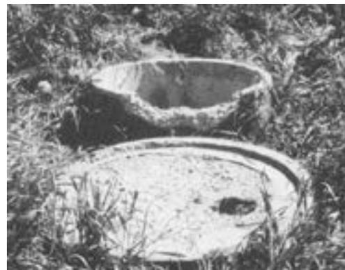
**Initial well-plugging steps include accurate measurement of the well dimensions and removal of all obstructions.**
