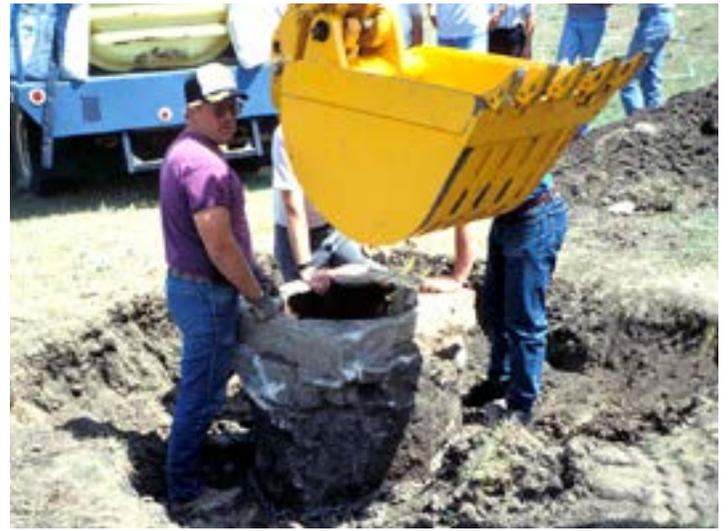
If the abandoned well site is intended for farming, removal of the upper 3 feet of the well casing after the abandoned well has been filled will eliminate the possibility of tillage equipment being damaged.
