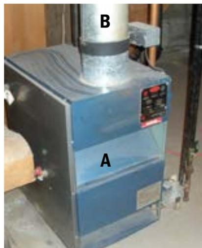
Draft inverter furnace. Note the large opening for intake air (A) and large galvanized pipe for exhaust air (B).
