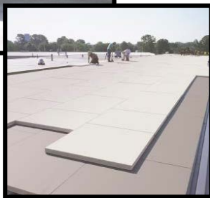
Figure 5. Continuous insulation on roof deck. (Courtesy of U.S. Department of Energy building codes university)
