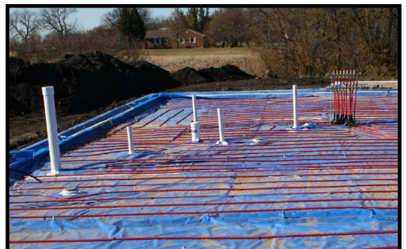
Figure 3. In-floor hydronic tubing. (Carl Pedersen, NDSU)
