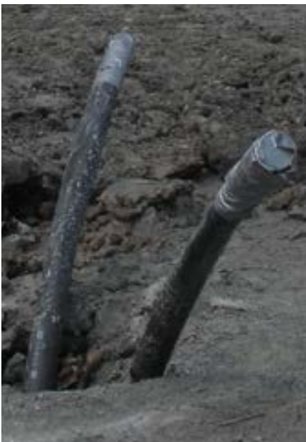
Figure 7. Installed vertical ground loop
