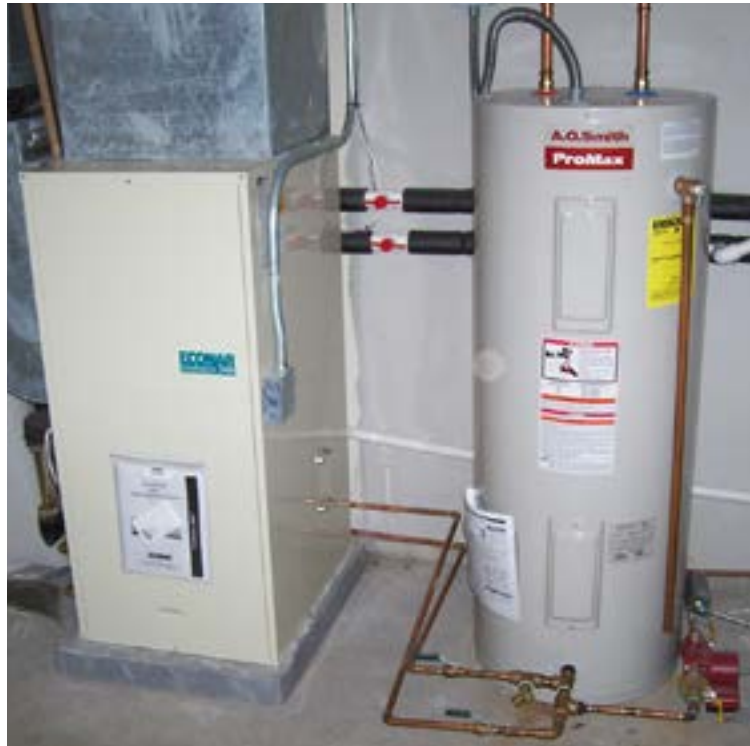
Figure 1. Forced-air heat pump with desuperheater.
