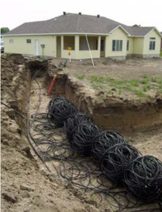
Figure 4. Horizontal “slinky” system installation (before)
