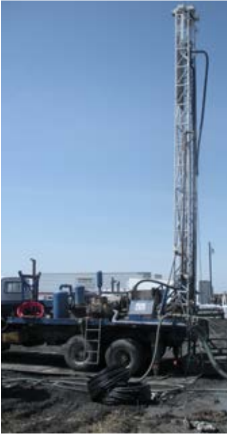
Figure 6. Drill rig installing vertical ground loop
