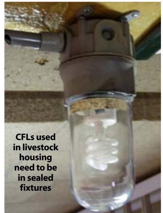
65 watt CFL replacement for 175 watt mercury vapor yard light
