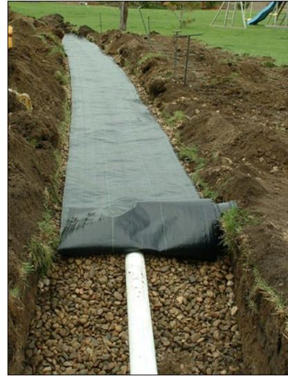
**Figure 13. Gravel-filled trench covered with geotextile fabric.**
