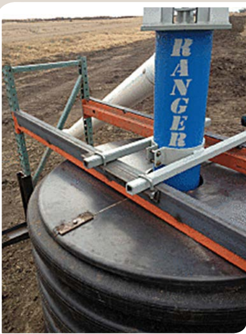
Figure 6. A metal frame is used to support the weight of a shaft-driven pump on a plastic sump casing.
