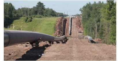
Laying Enbridge pipeline in ND.
