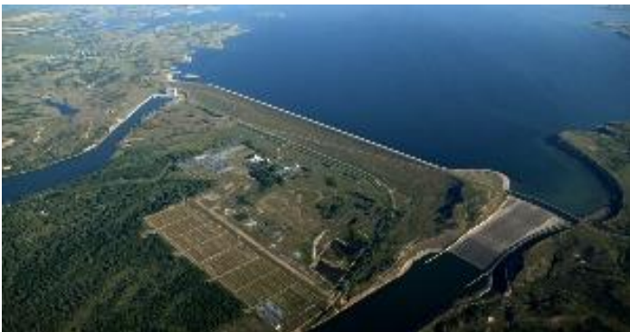
Garrison Dam in central North Dakota is two miles long.
