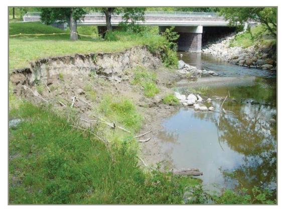
Figure 21. An example of bank erosion, courtesy of Red River Riparian Project, 2011.
