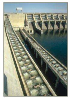
*Figure 67. This photo shows fish ladders along a dam, courtesy of the U.S. Army Corp of Engineers, 2012.*
