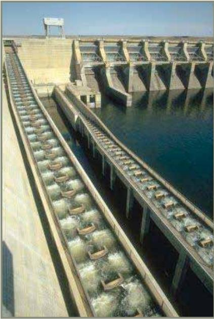
Figure 67. This photo shows fish ladders along a dam, courtesy of the U.S. Army Corp of Engineers, 2012.
