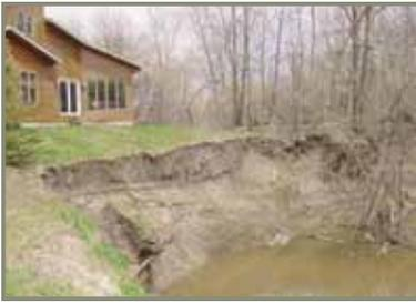
Figure 24. Extreme riverbank erosion likely caused by the lack of native vegetation and frequent mowing to the edge, courtesy of Red River Riparian Project, 2012.
