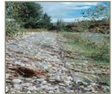
Figure 37. A photo showing the use of riprap along a stream, courtesy of Cows and Fish, 2012.
