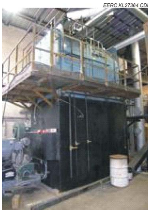
Figure 9. King Coal stoker for combustion of coal or wood (King Coal Furnace Corporation, 2006).
