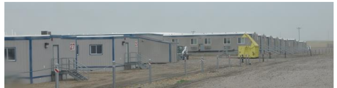
This man camp located near Tioga can hold 1,200 people.
