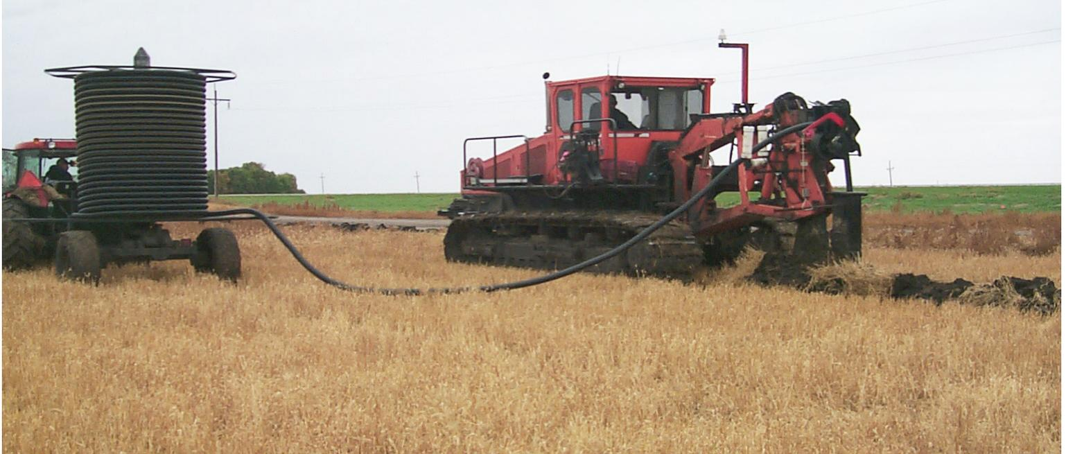
**Figure 11. Installation of tile drainage in progress in Ramsey County along state Highway 17 near Edmore, N.D. (Photo courtesy of Ronald Beneda, NDSU Cavalier County Extension agent).**
