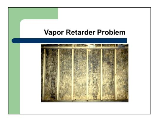
This shows mold growing on the oriented strand board in a wall. This view is looking at the wall from inside the house after the wall was opened and the insulation was removed. The polyethylene vapor retarder was improperly installed, which permitted air from within the house to enter the wall cavity near the ceiling. Moisture condensed on the exterior wall surface creating a wet environment that permitted mold growth.
