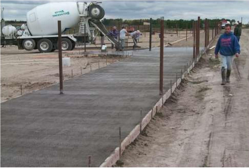
**Placing the fly ash/bottom ash aprons at the bison research facility, CREC.**
