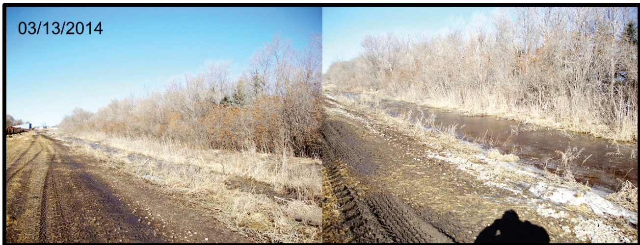
Figure 1. View of the clean water diversion system during later 2014 winter. The structure is located on the north and east side of the feedlot (partially seen on the left photo).
