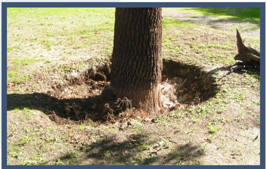
Sediment deposited can suffocate roots and lead to long term health problems of trees.
