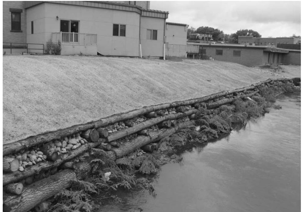
The tour of southeastern North Dakota included a stop to see a riparian log crib wall on an erosion control project along the Sheyenne River in Valley City.
