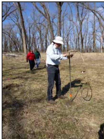
Preparing 6-foot deep unrooted cutting hole with water jet stinger
