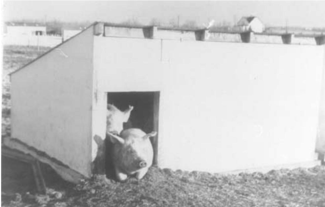
These hog houses, 10 feet by 8 feet are of wood construction with a metal roof. The sills are 4 inches by 4 inches firmly braced to be used as runners. The cost of each building was about \$80.00.
