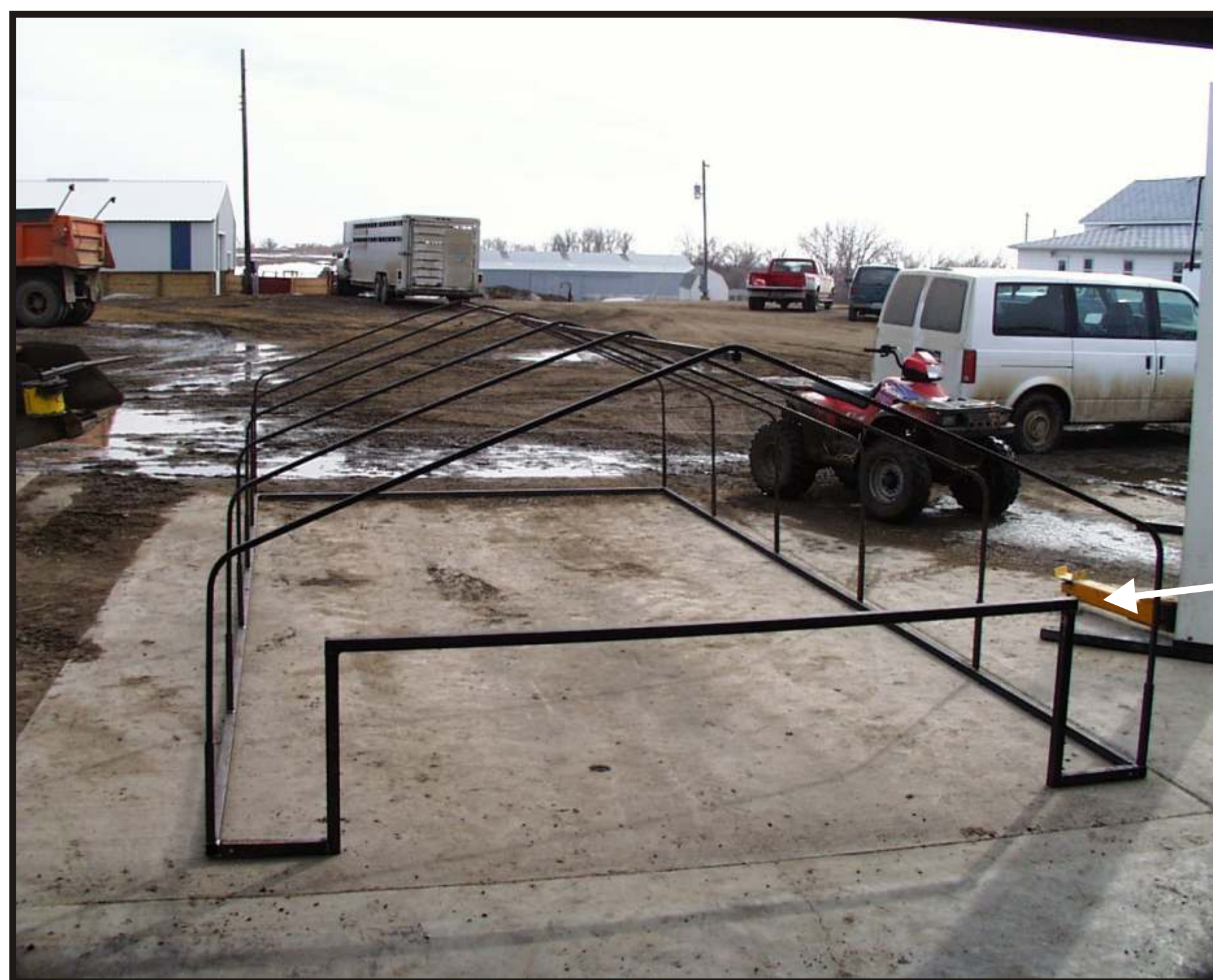
Figure 6. Finished frame. The hoops are spaced 5' apart and will be covered with white metal siding.
