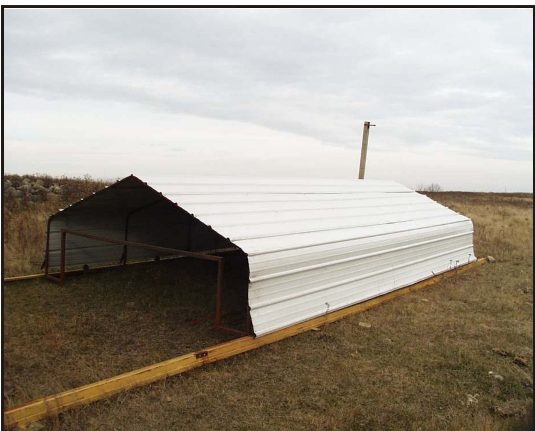
Figure 7. The shelters are covered with steel siding similar to material used on metal pole buildings.
