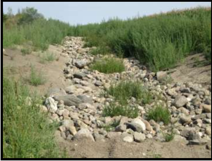
The end of the diversion ditch is rocked to reduce erosion.
