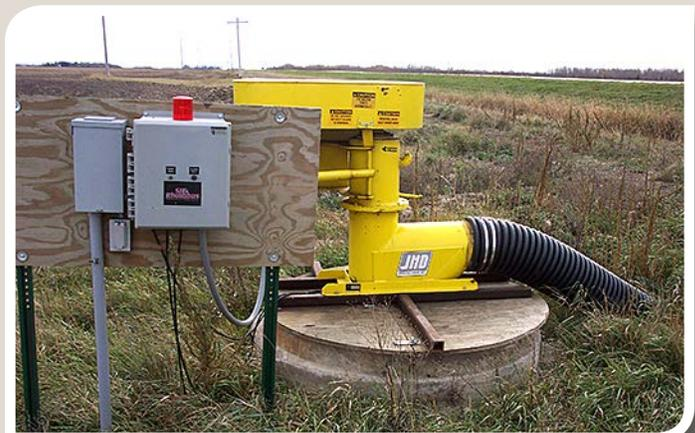
**Figure 4.** A concrete casing with metal cross beams supports the weight of the pump in this drainage lift station. This lift station also has a wooden cover with an access door. (NDSU photo)
