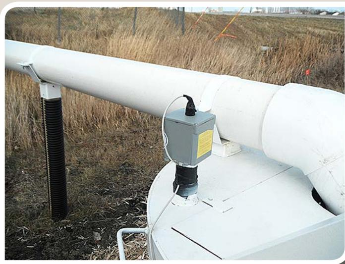
Figure 10. A pressure transducer box and pipe are part of this VFD-controlled pump. (NDSU photo)
