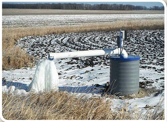
**Figure 3.** This drainage lift station uses a manufactured plastic sump casing with a metal cover containing a submersible pump. This photo was taken in mid-November when the temperature was below freezing. (NDSU photo)
