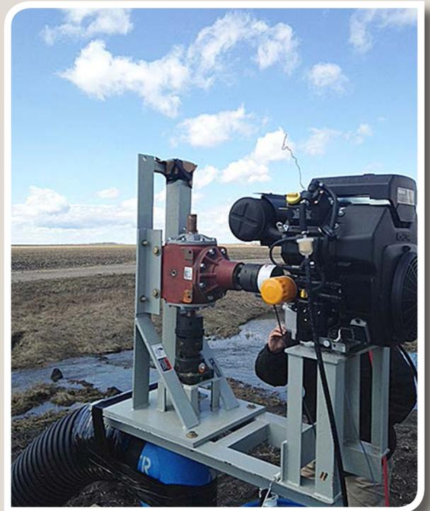
**Figure 14. This engine powered drainage lift pump is controlled by water level sensors in the sump.**
