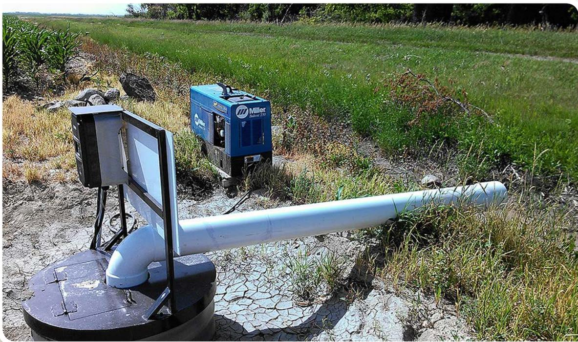
Figure 13. A generator is used to power the VFD-controlled submersible pump in this drainage lift station.
