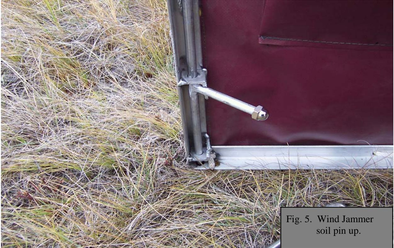
Fig. 5. Wind Jammer soil pin up.
