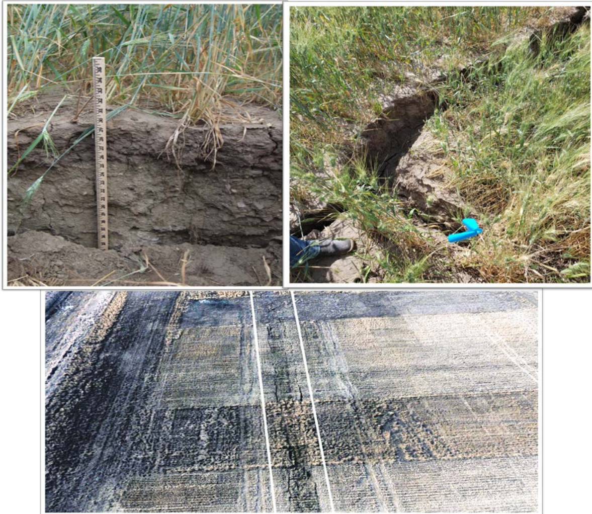
Figure 6. Images of subsidence along the pipeline disturbance area. The upper two images were taken after the subsidence occurred in July 2018. The aerial image was taken in March of 2019, the sunken area is outlined in white.
