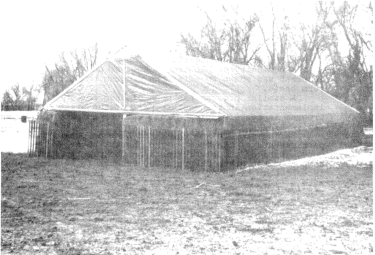
A SHED MADE FROM STRAW USED FOR A SHEEP SHELTER
